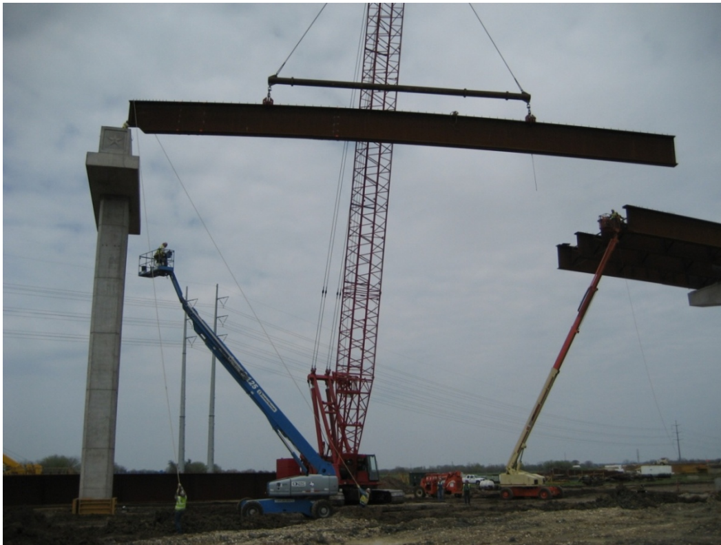
Figure 3.4 Girder 4 Lifting
