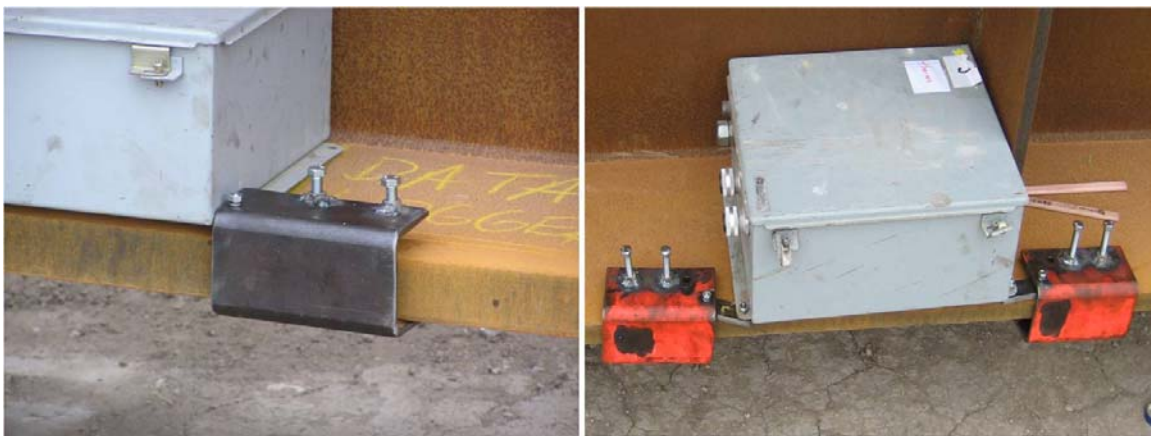
Figure 2.14 Metal Boxes Attached To Girder Flange
