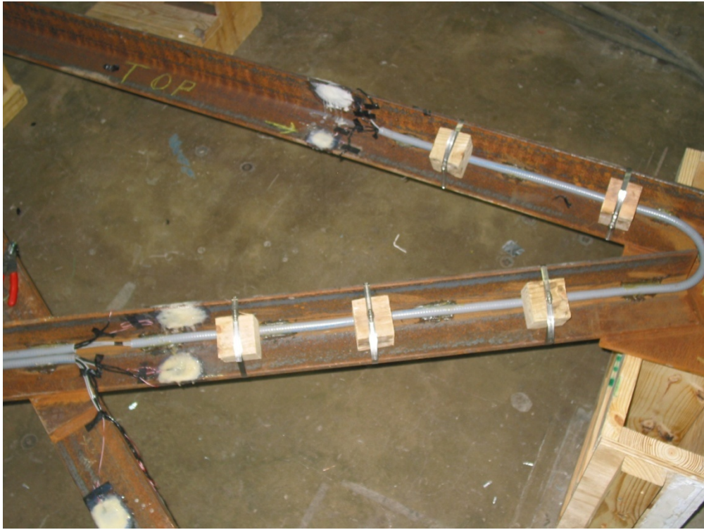
Figure 2.11 Conduit Braced w/ Wood Blocks on Cross Frame
