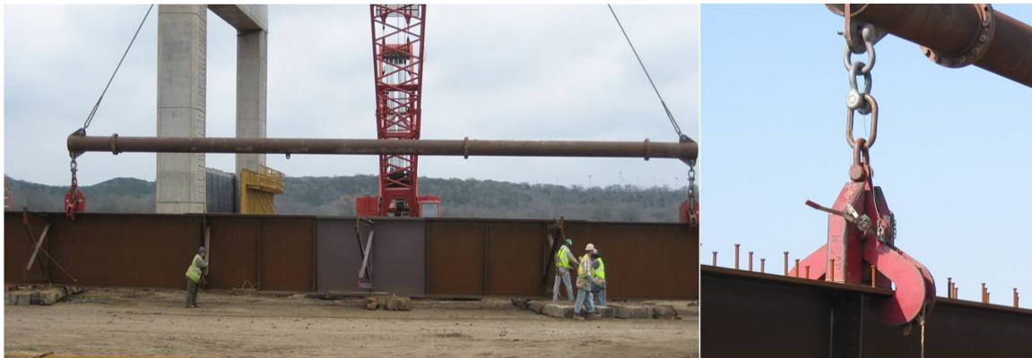
Figure 3.1 Spreader Bar and Lift Clamp Apparatus
