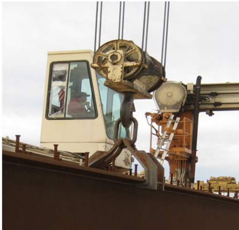
Figure 3.28 MI-JACK Lift Clamp Apparatus
