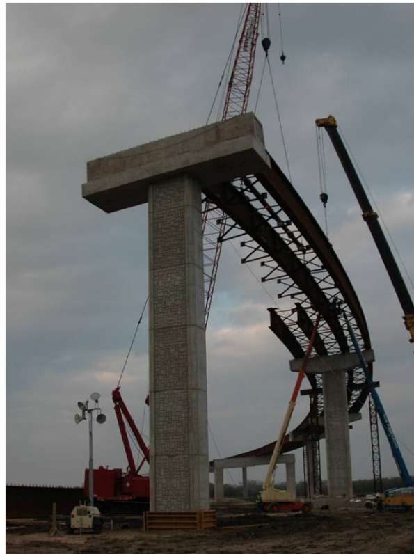
Figure 3.8 Erected Girder 4 & Girder 3 of Span 14-Unit 6
