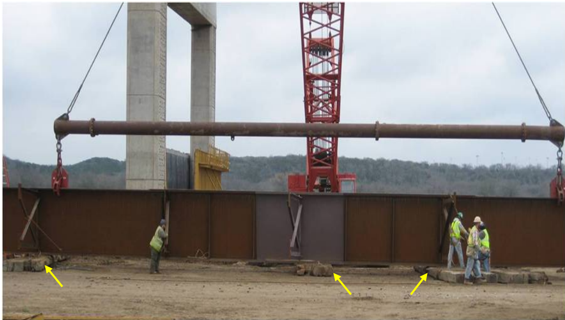
Figure 3.25 Dunnage Used for Girder Support
