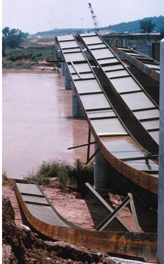
Figure 1.2 Girder Instability
