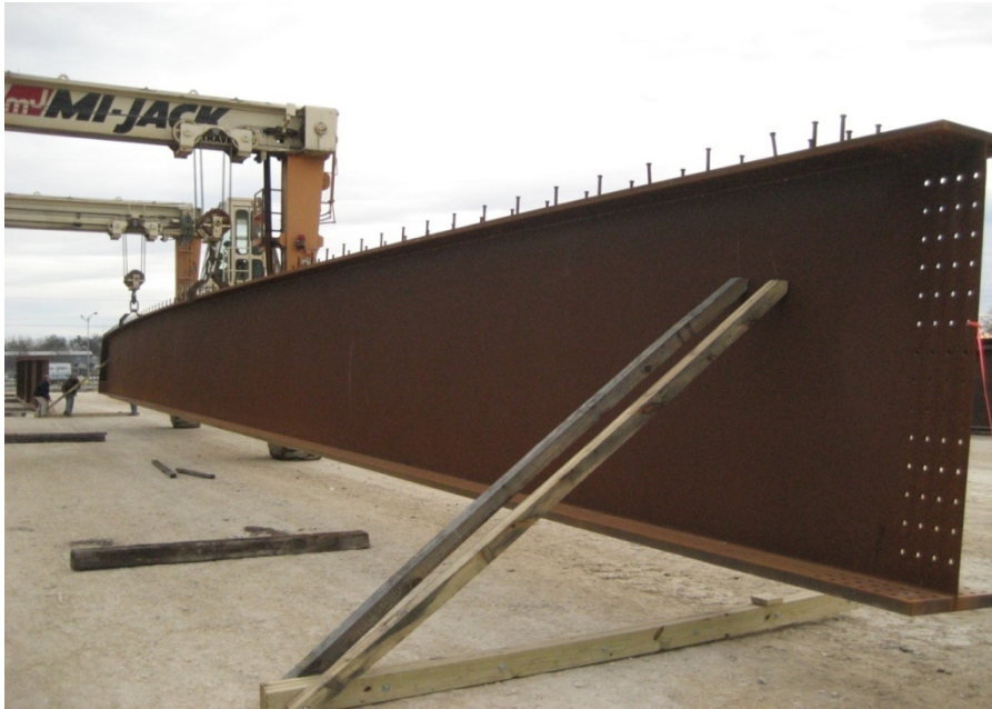
Figure 3.31 16C4 Lifted at S1 (8:30)
