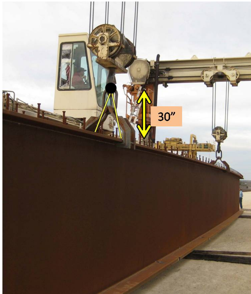
Figure 4.3 Lift Apparatus and Axis of Rotation Location
