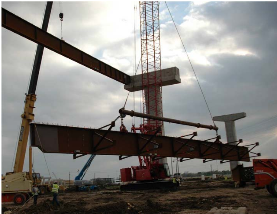
Figure 3.7 Girder 3 and Cross Frame Lifting
